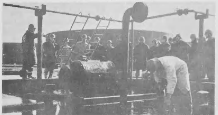
Well protected by fog spray, Marines replace broken ball in overhead leaking flange.
